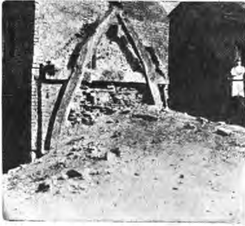
FIG. 34.—Photograph of a demolished house with the old crucks built about with new walls.
